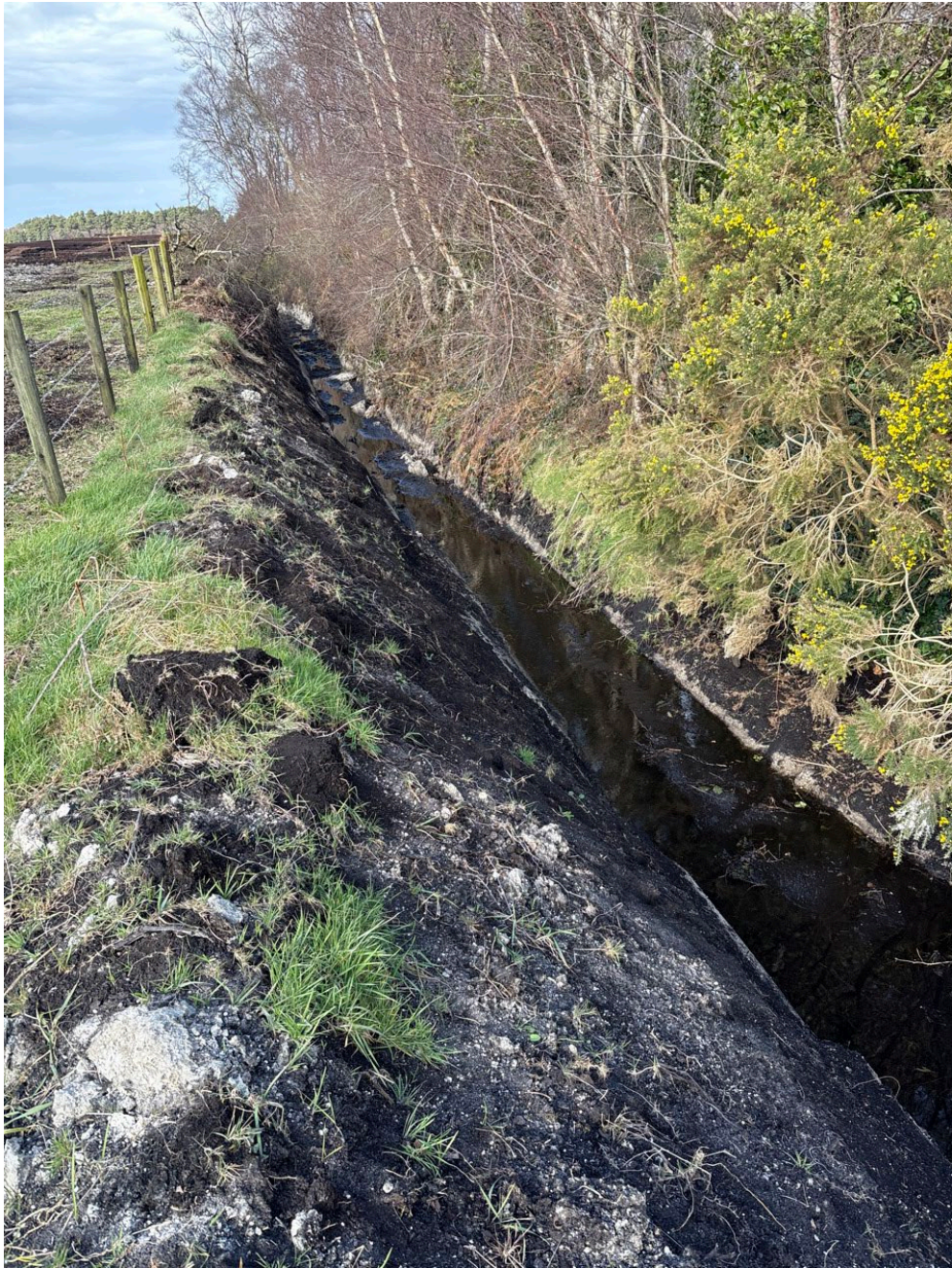
Deep land drain crossing T3 hardstanding area and access track
